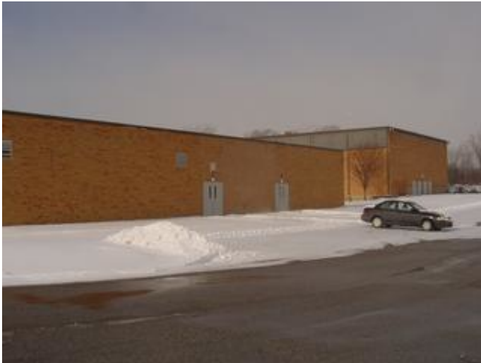
South elevation photo:
