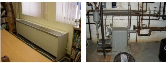
Heating system is boiler system linked to unit ventilators. Does not provide required CFM and gym heating system original 1923 system. Limited AC provided in the building
