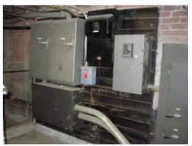
Electrical system in poor condition, and not of adequate capacity
