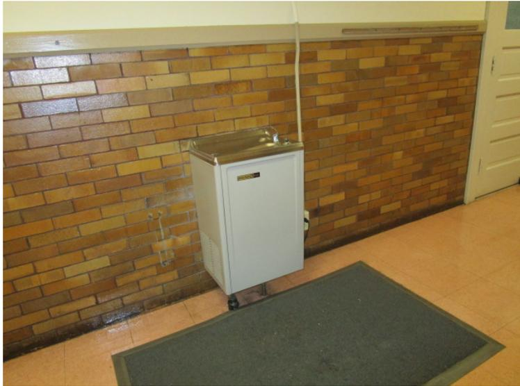
The building violates many ADA requirements. Although an elevator has been added to this 2 story but 5 level facility many other ADA requirements are lacking such as ADA door hardware throughout, ADA water coolers, ADA signage, etc.
