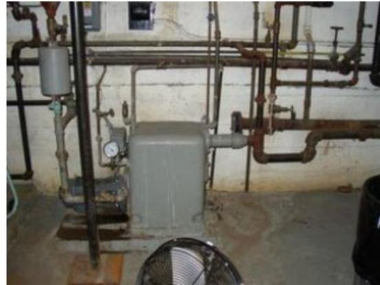
Heating system is boiler system linked to unit ventilators. Does not provide required CFM and gym heating system original 1923 system. Limited AC provided in the building
